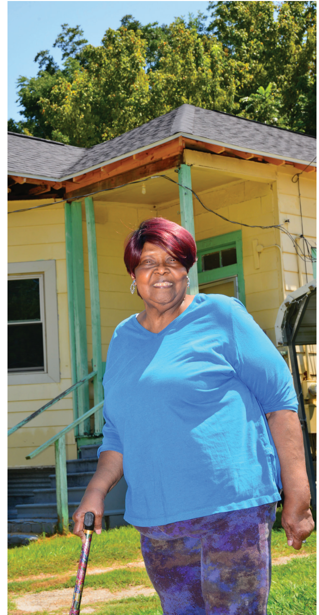
Ethel Franklin has a storm-resistant roof thanks to a $15,000 FHLB Dallas FORTIFIED Fund grant through RiverHills Bank.
